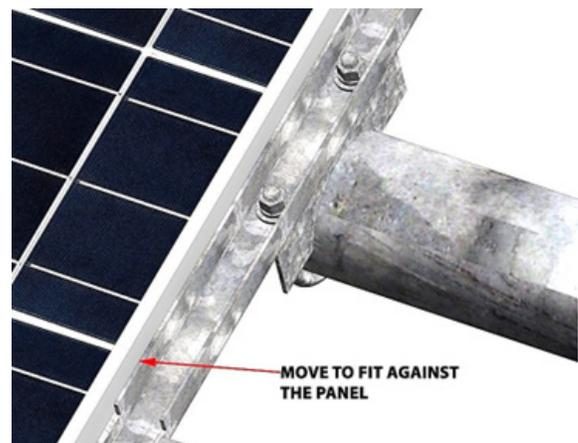
Loosen the End Clamp U-Bolts if necessary and move it to fit firmly against the solar module frame and re-tighten to hold position.
